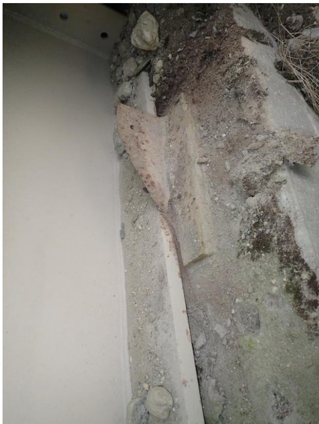
Figure 22: Right abutment girder 1 bearing upstream face - note bearing against restraint.
