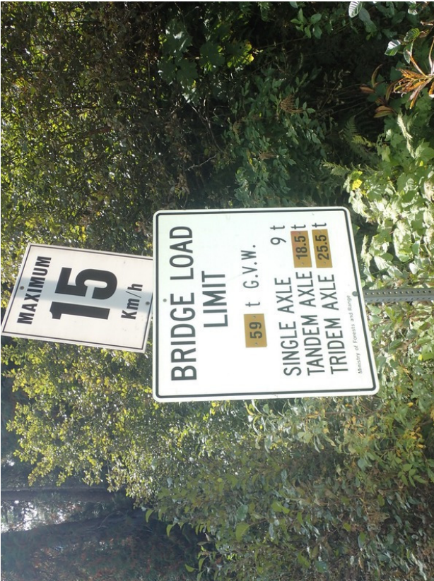
Figure 6: Load posting and speed limit signs at right approach.
