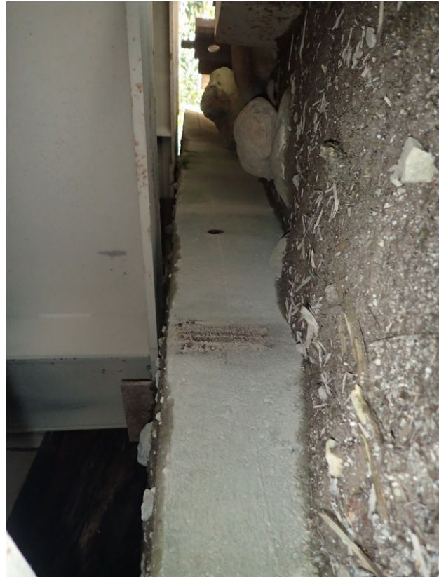
Figure 28: Left abutment concrete sill.
