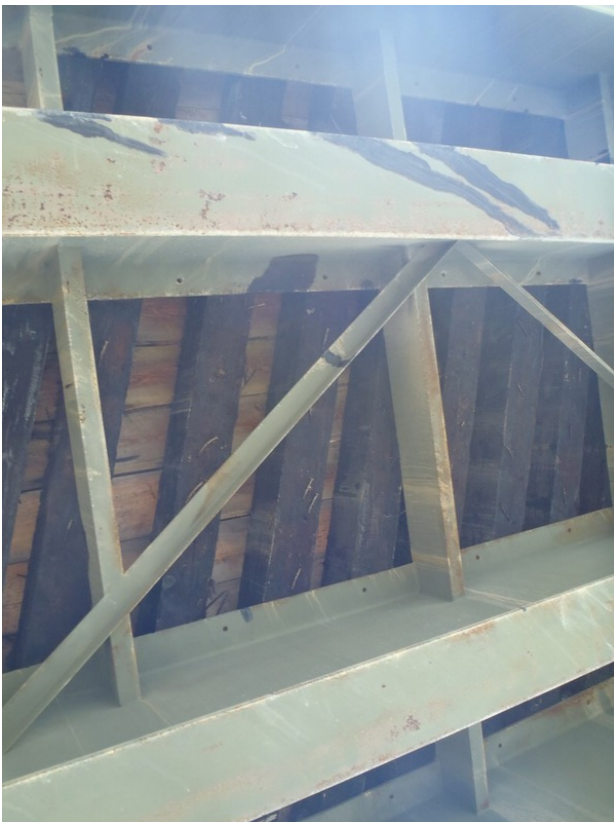
Figure 13: Typical sub deck condition.
