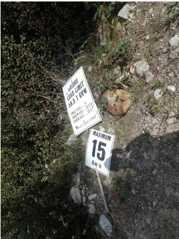
Figure 9: Load posting and speed limit signs - left approach.
